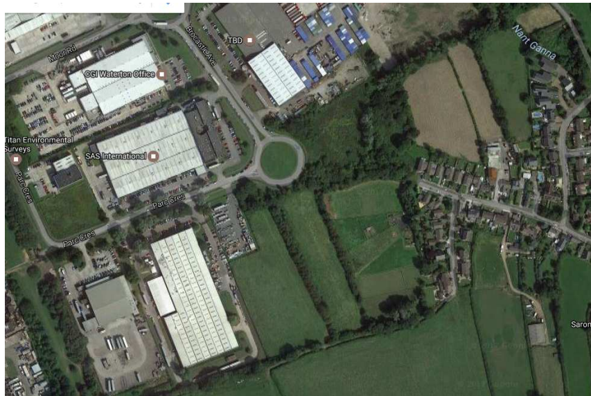
Fig. 3: Aerial Photograph of the site
